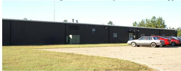
50,000 SF metal building consisting of 30,000 SF manufacturing area, 10,000 SF air conditioned warehouse/office area, and 10,000 SF non-air conditioned warehouse. The finished  $150 \times 200$  manufacturing area has three rows of interior columns with  $33 \times 50$  bays.
